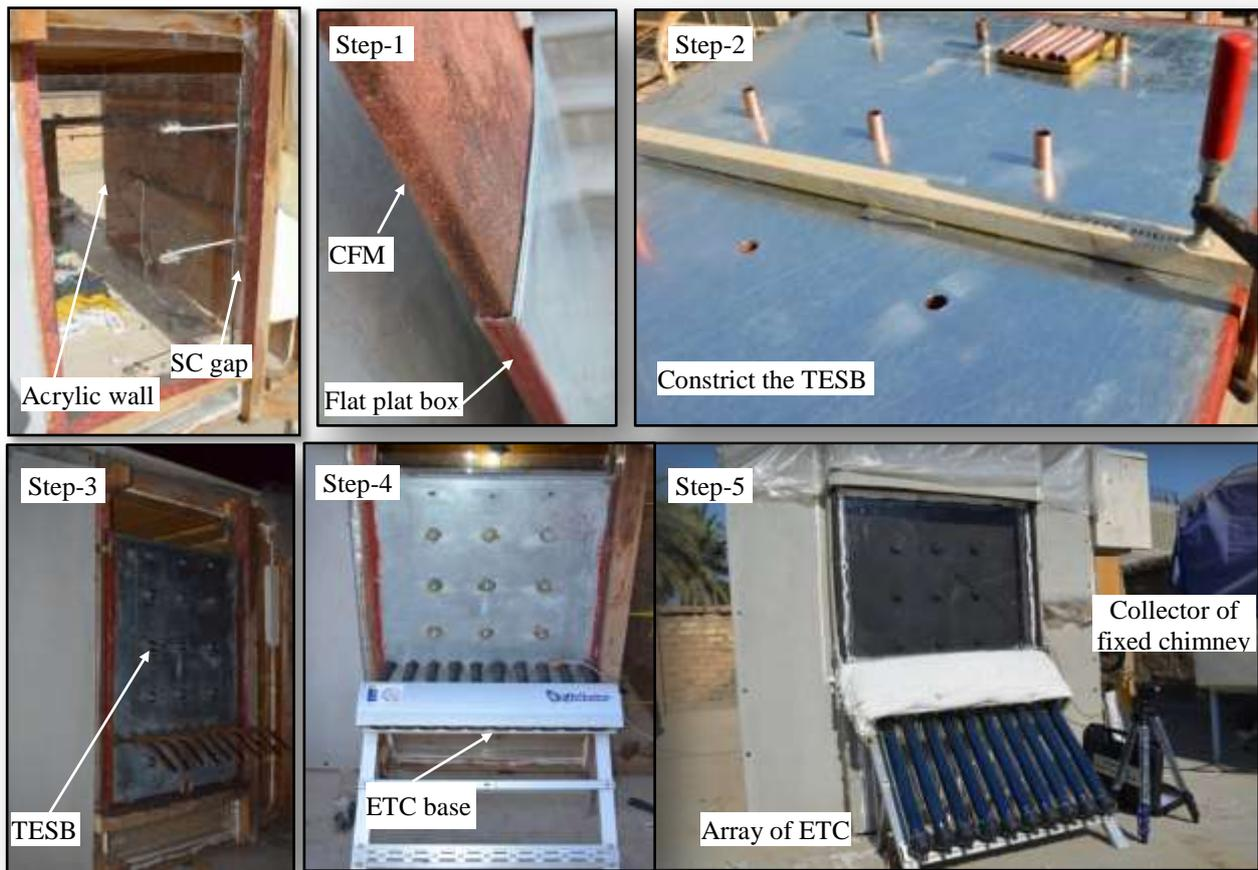
Fig . 5 Stages to manufacture the vertical fixed SC and setup in the test room.
