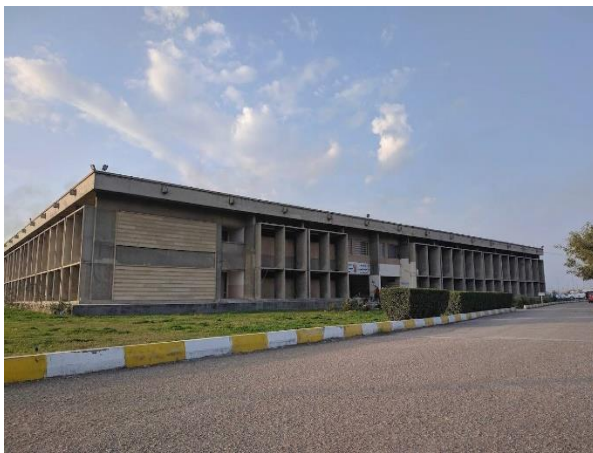
Fig . 1. Lecturing building of Al-Khwarizmi College of Engineering.
